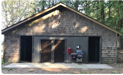
Main Camp Bathrooms & Showerhouses
